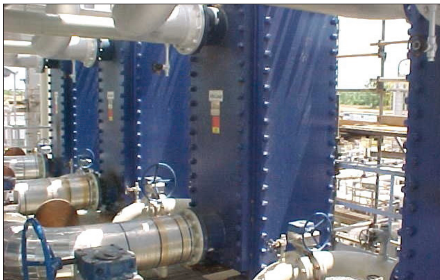
Figure 8 CPHE installation for recovery of a total of 14 MW from FCC overhead vapours into BFW loop.
