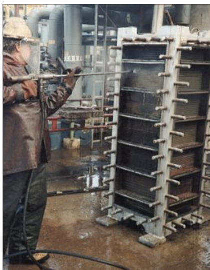
Figure 4 CPHE provides unrestricted access to the heat-transfer surface for mechanical cleaning
