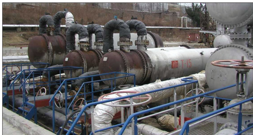
Figure 3 Difference in heat-transfer area and ground space for a S&T compared with a CPHE installation in a heat-recovery installation (atmospheric residue: 288 →162°C; crude:107 → 201°C; heat load: 7MW). S&T total heat transfer area is more than 1000 m 2 and CPHE heat transfer area area is only 170 m 2
