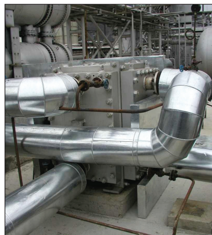
Figure 3 Difference in heat-transfer area and ground space for a S&T compared with a CPHE installation in a heat-recovery installation (atmospheric residue: 288 →162°C; crude:107 → 201°C; heat load: 7MW). S&T total heat transfer area is more than 1000 m 2 and CPHE heat transfer area area is only 170 m 2
