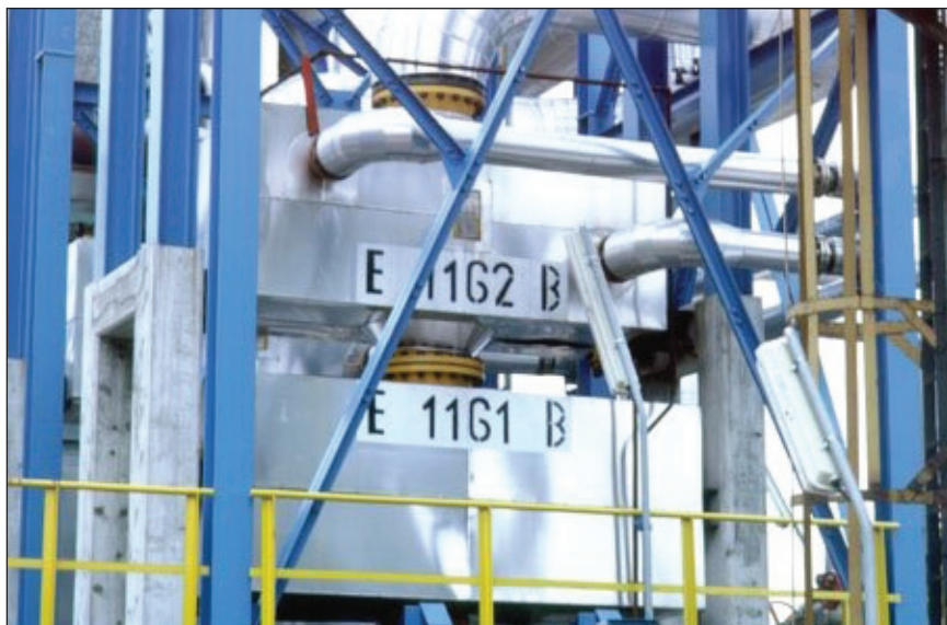
Figure 6 One of the two CPHE pairs mounted on top of each other for preheating BFW and crude by means of naphtha toppings
